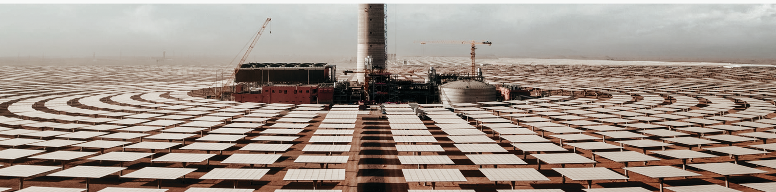
The Noor III Concentrated Solar Power (CSP) tower, Ouarzazate, Morocco. Uses molten salt storage to supply electricity after sunset, showcasing utility-scale renewable energy in arid, climate-vulnerable regions. (ArcelorMittal, 2018. Source: Noor III – ArcelorMittal Europe News)
